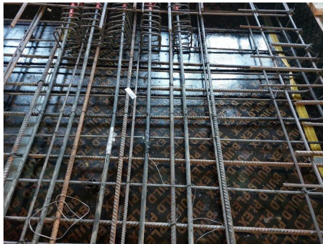
Figure 6. installation of tendons' strain gauge
