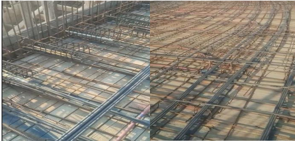
Figure 3. Unbonded post tension slab
